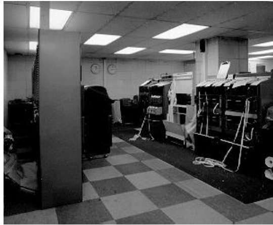
Line Room in the East Block
